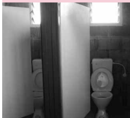
The new 'pink house' toilet blocks offer a hygienic facility to the girls.
